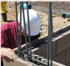
**Location of Reinforcing Steel and Joint Reinforcement**
